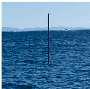
Fig. 5. (A) Photo of half of the fixed platform (i.e. three 4-m legs and three cross members.) (B) Drawing of the fixed platform including the legs, cross-members and helical anchors. (C) Photo of the installed submerged platform with a navigation light ~2 m above mean sea level.
