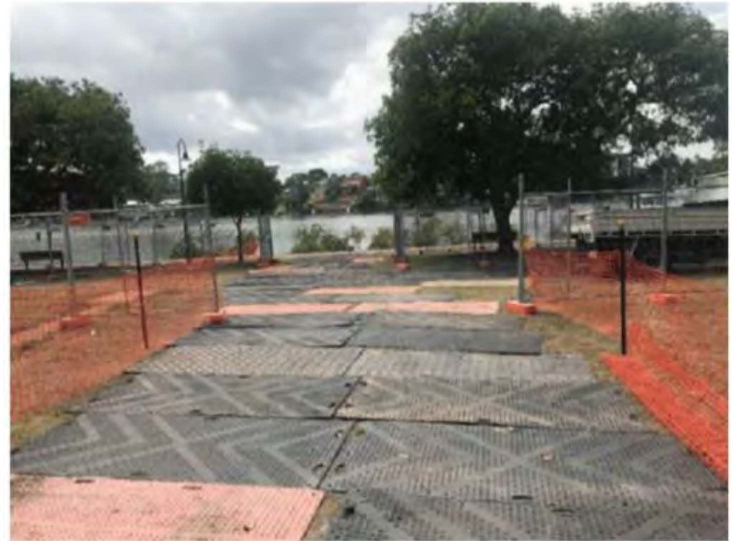
Figure 6: Ground Protection Mats (source: Arbor Australis)
