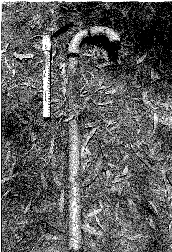
Figure A.46 : Antenna stay anchor attachment.
