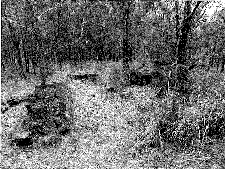
Figure A.43 : Concrete anchors removed from original positons in the ground.
