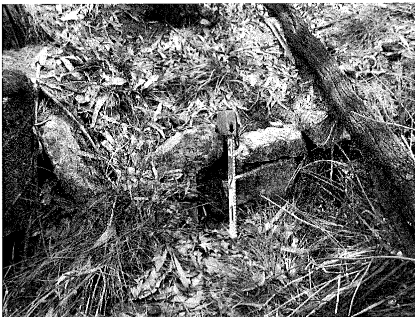
Figure A.49 : Stone lined drain alongside access road, north of main building. Concrete culvert left of image.
