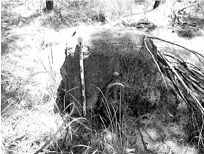
Figure A.45 : Concrete anchor and stay attachment removed from original position in ground.
