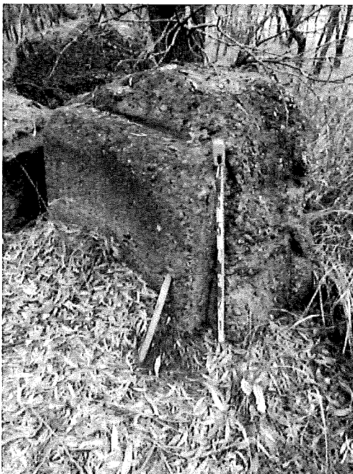
Figure A.44 : Concrete anchor and stay attachment detail.
