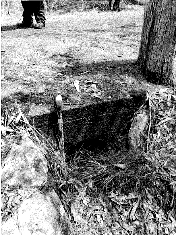
Figure A.48 : 1940s era concrete culvert with stone lined drain, north of main building.
