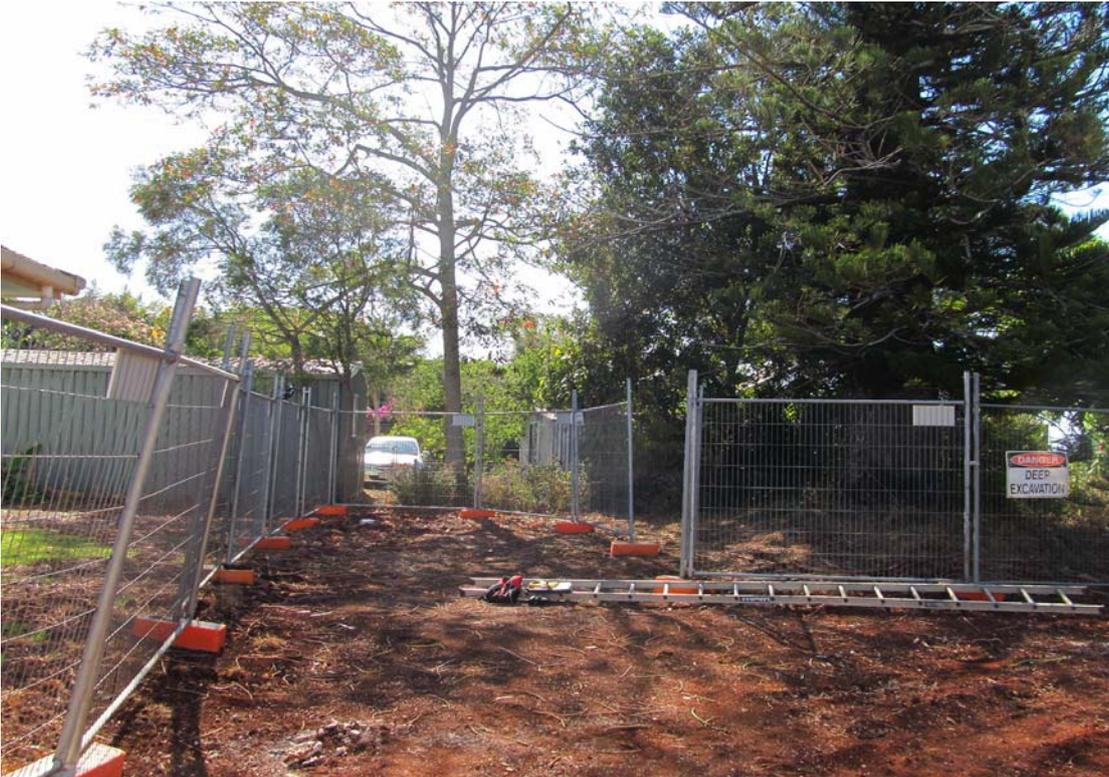
**Figure 7:** Photograph - Sewer trenching occurred 7 metres from the trees trunk and can be seen in the photo as a white inspection cap near the white car. The exact sewer alignment is unknown but appears to be outside the structural root zone.
