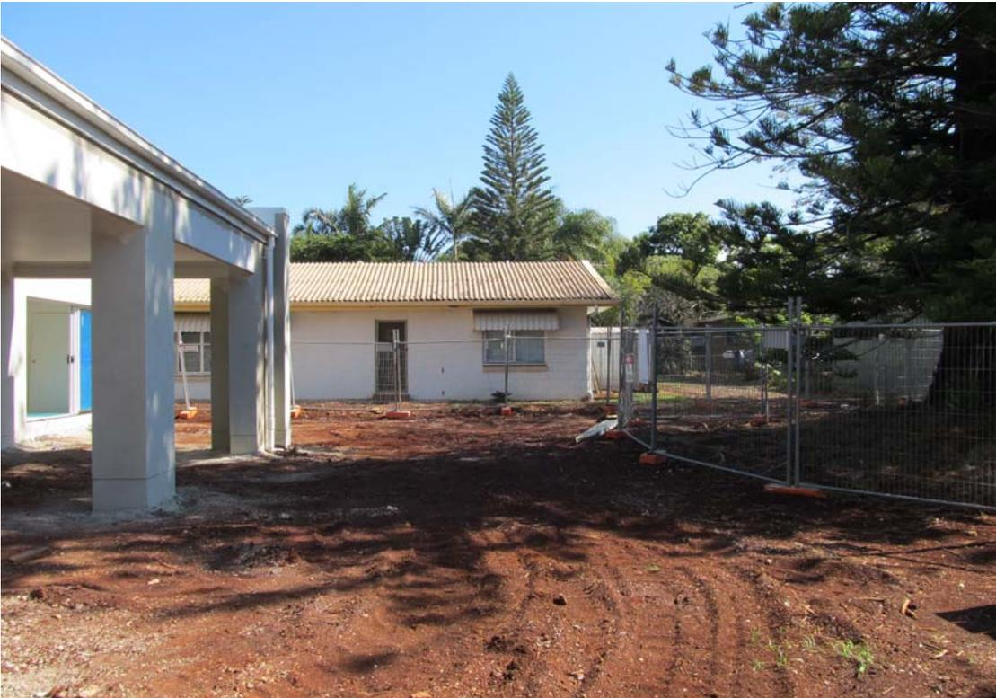
**Figure 8:** Photograph - Looking west. There will be a 3 metre wide concrete pad constructed from the house pillars towards the tree. The distance from the concrete to the tree will be 6 metres.
