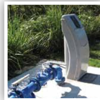
New electronic filling station for use by potable water carriers at Valley Way, Mount Cotton.
