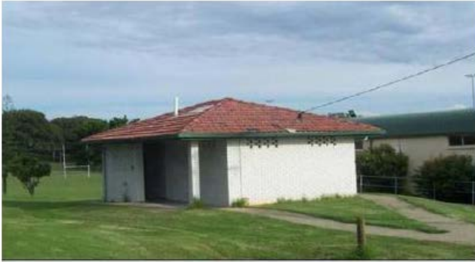
Image 1 – Dunwich public toilet block with clubhouse in the background
