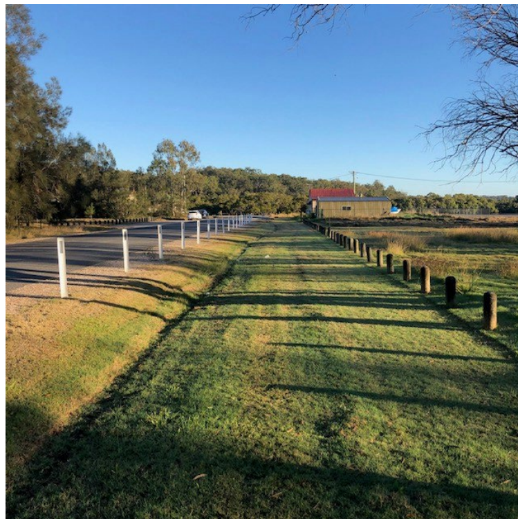
Open roadside vegetated swale at Railway Parade filters and calms water.
