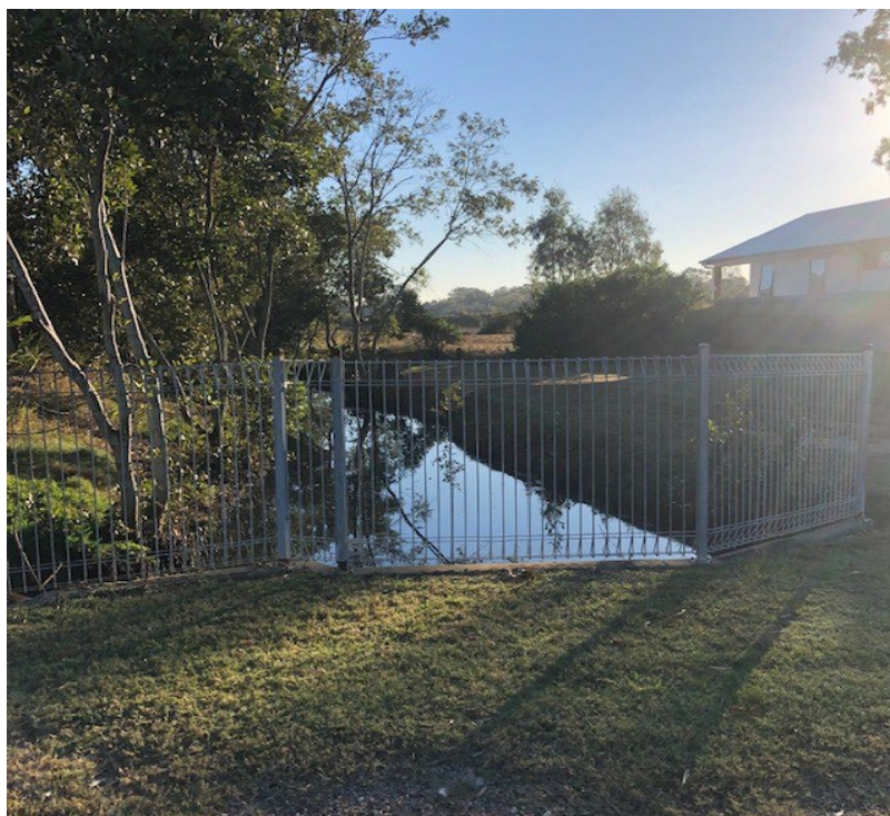
Drainage channels crossing Ferry and Thorneside roads.
