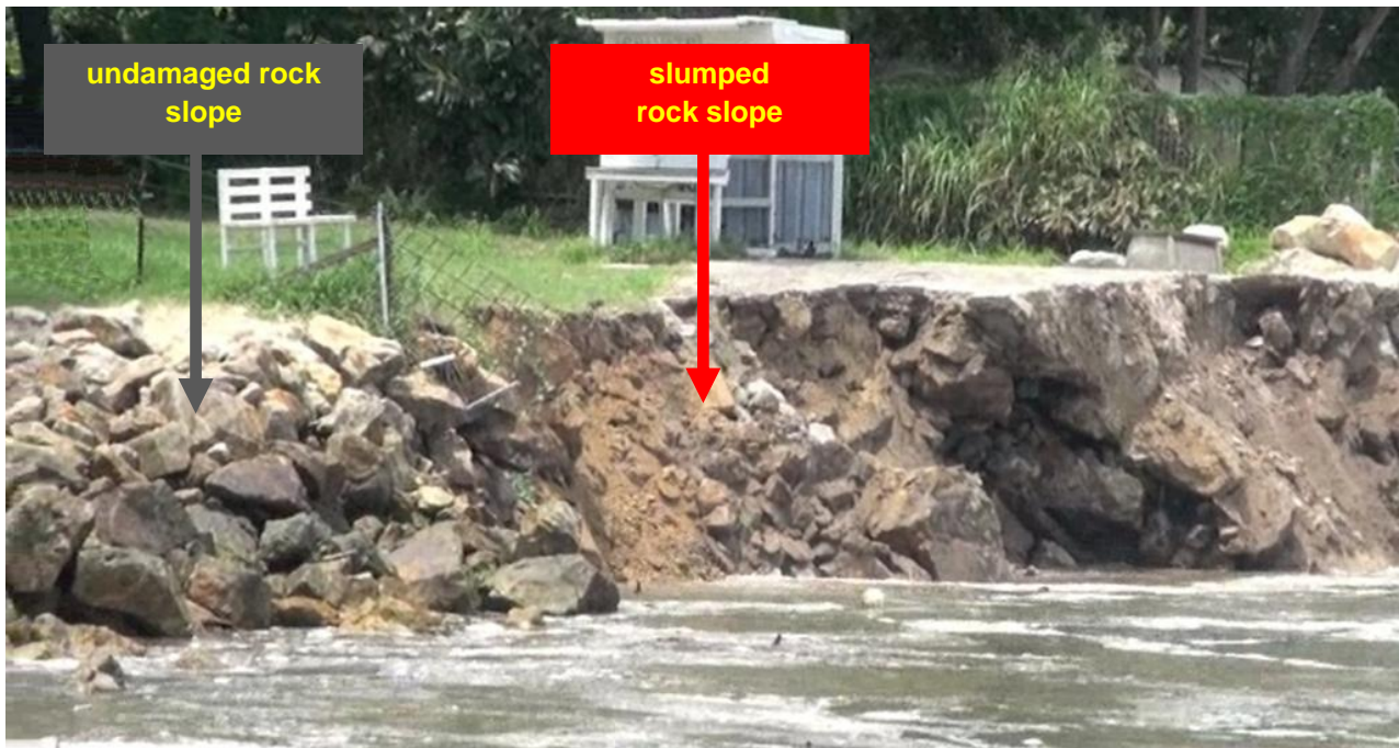
Figure 3-1 Emergency Tidal Works Trigger Event – Excessive Rock Slumping
