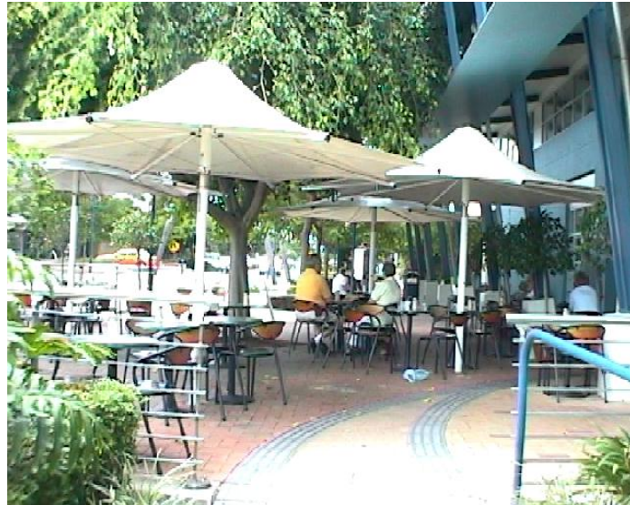
Photograph 6 - Tactile paving free of obstructions
