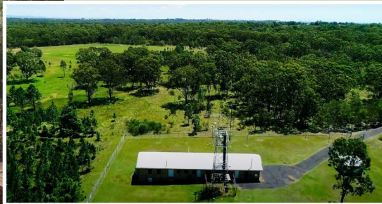
Former World War II Radio Receiving Station
