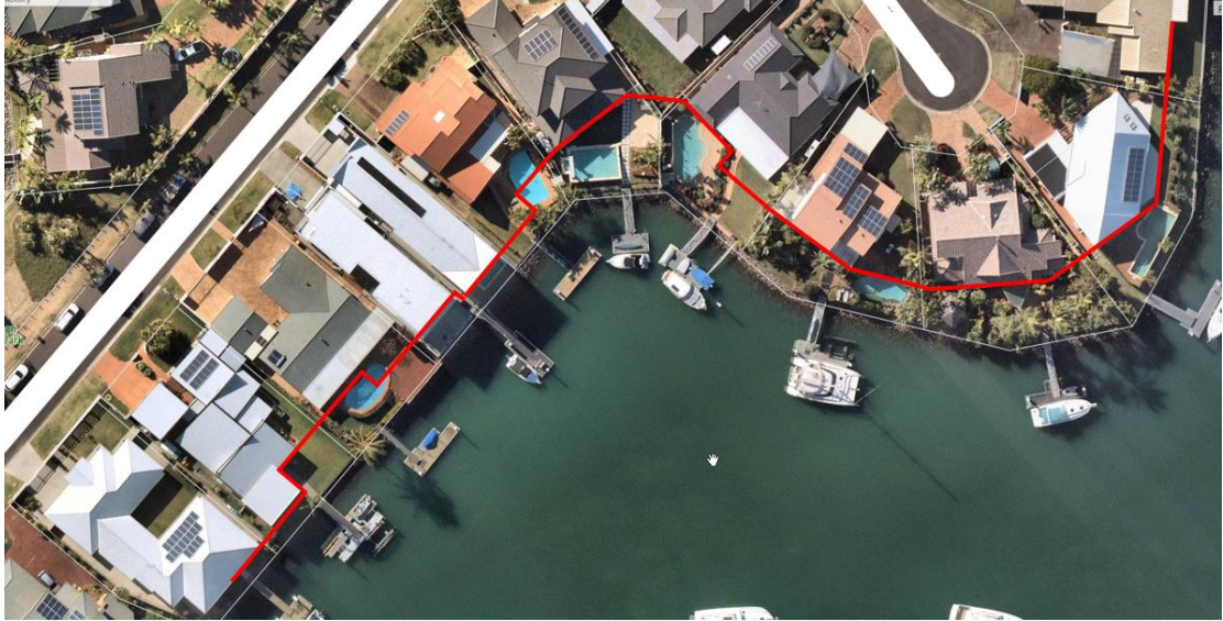
Figure 6.2.1.2.7 - To achieve compliance with PO9, dwellings may develop closer to the canal/lake, up to the red line. The centre of a site is used to delineate the location on the site where the red line changes to reflect the setback of the adjoining dwelling.
