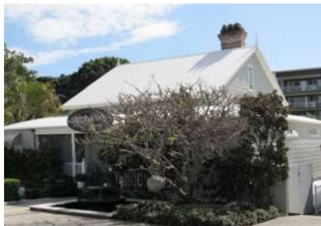
Residence, 200 Middle Street, Cleveland (RPS, 2012).
