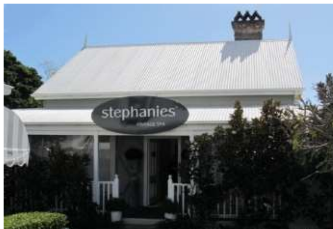
Residence, 200 Middle Street, Cleveland (RPS, 2012).
