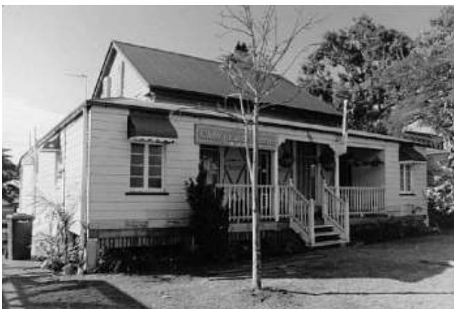
Residence, 200 Middle Street, Cleveland (RPS, 2012).
