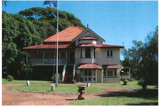
Somersby Grange, Birkdale (EHP, 2009).
