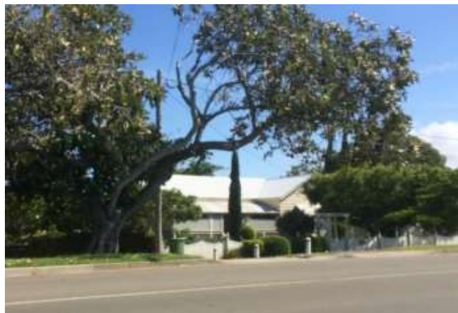
Residence, 19 North Street, Cleveland (AHS, 2017).
