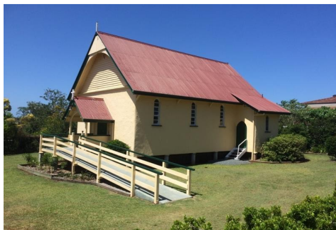
St James' Anglican Church, Wellington Point (AHS, 2016).
