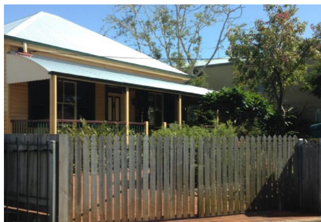
Residence, 17-18 Esplanade, Wellington Point (AHS, 2017).
