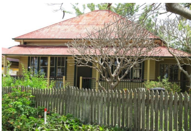
Residence, 17-18 Esplanade, Wellington Point (RCC, 2012).
