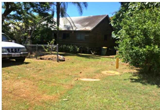
Residence, 11 Parsons Street, Dunwich (AHS, 2016).
