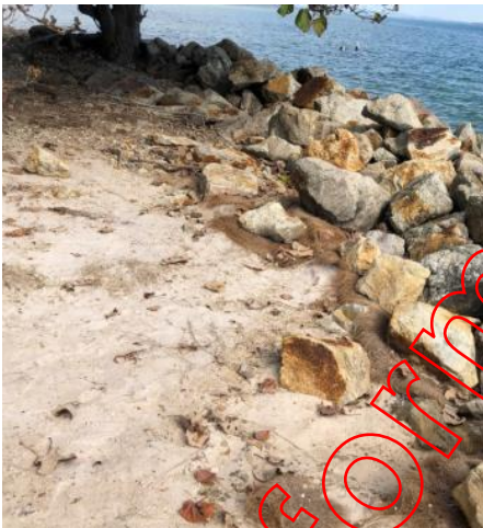
(c) sea wall crest
