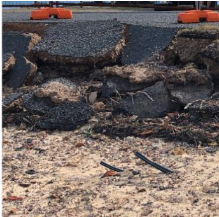
(a) bitumen erosion from tide
