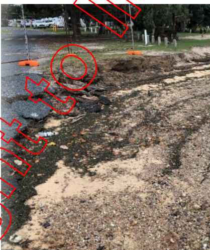
(e) Bitumen seal cracking along the beach
