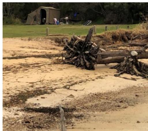
(f) Park Beach (gravel from road base on the beach)
