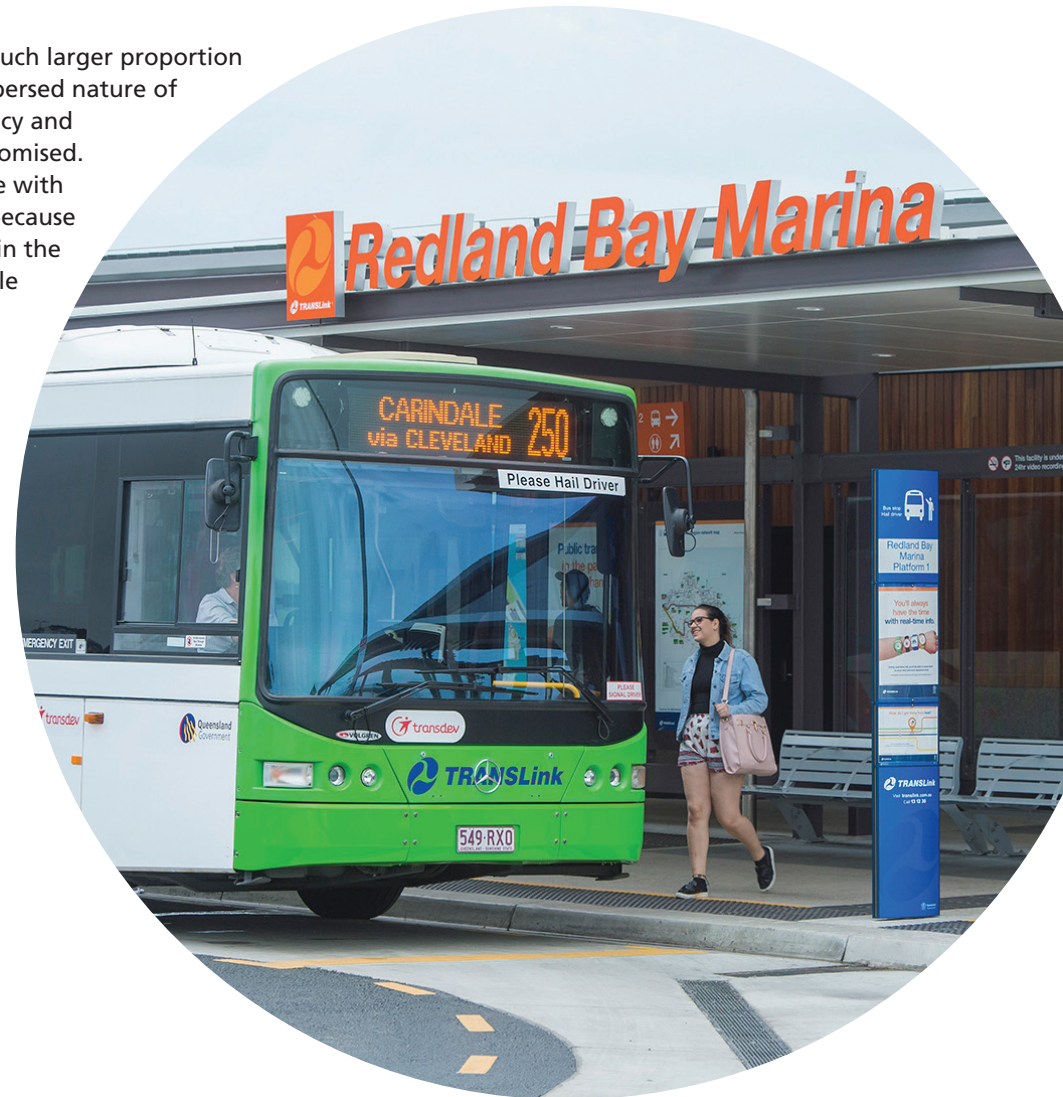
Redland Bay Marina bus interchange
