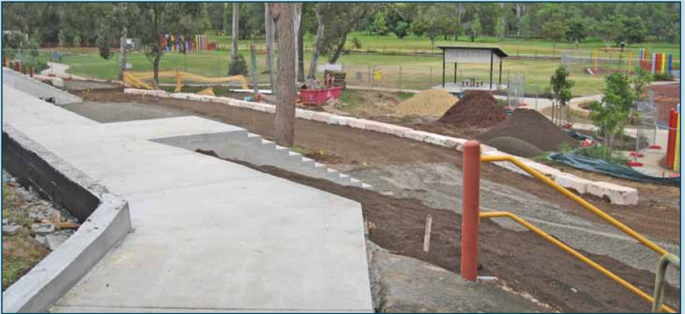
Works underway at Capalaba Regional Park.
