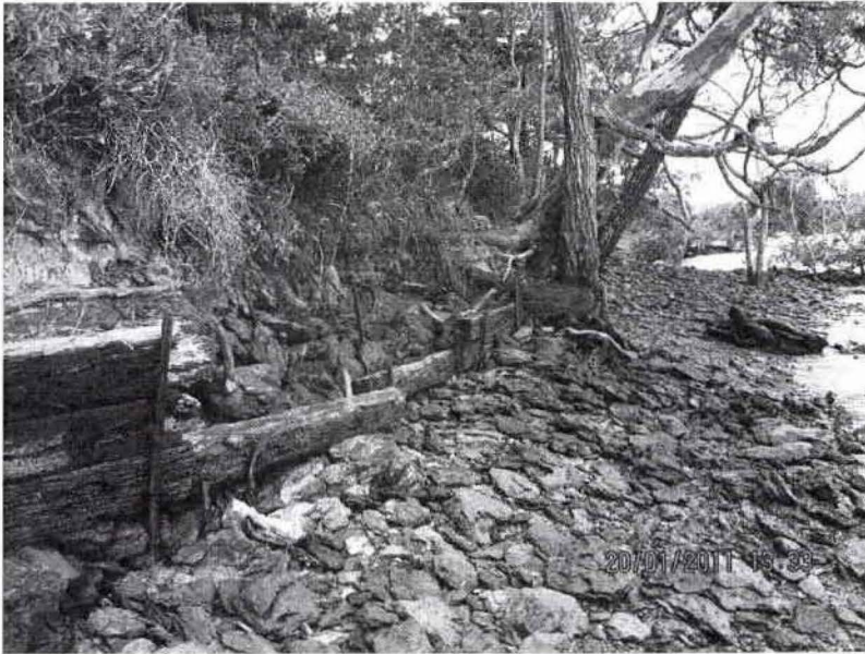
Figure 4 Wooden seawall facing east along the foreshore
