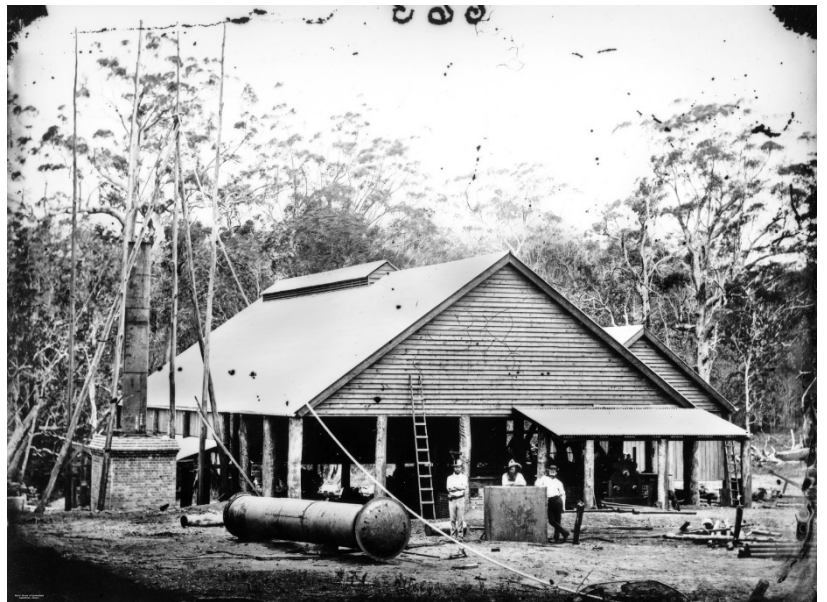
Workmen taking a break from raising a chimney at the sugar mill, c1871 State Library of Queensland
