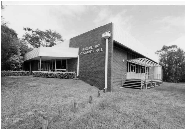
Redland Bay Community Hall c2004 HP4568
