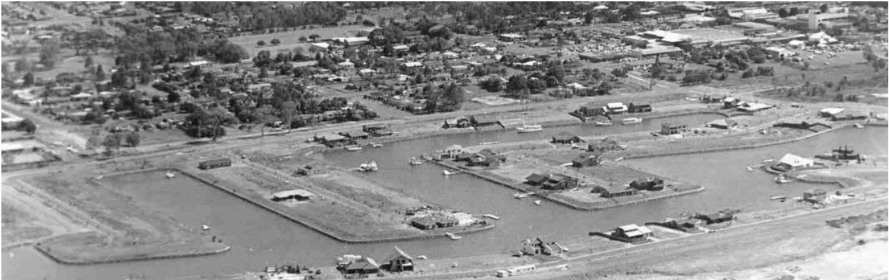
Raby Bay canal estate under construction, mid-1980s
