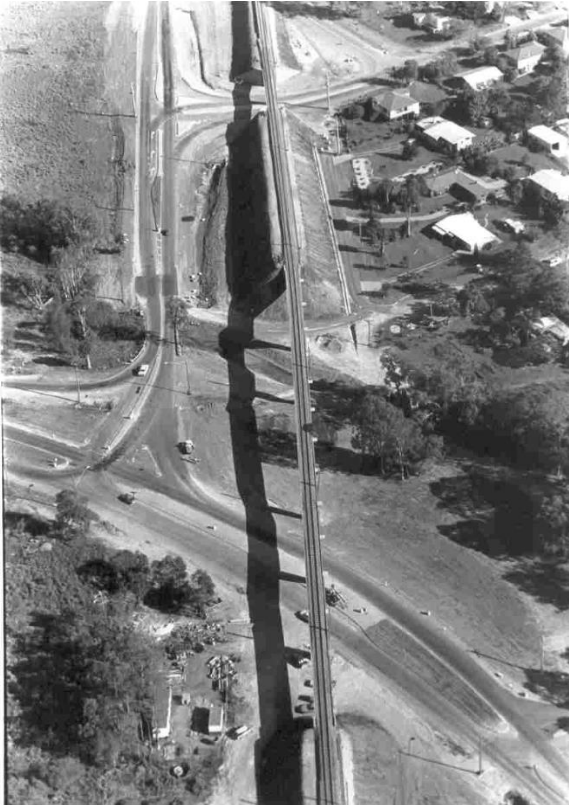
Aerial image of the 1986 railway overpass on Birkdale Road.
