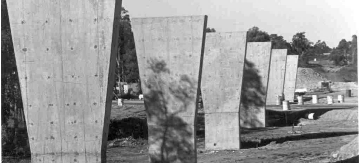
Railway overpass under construction for the Thorneside-Wellington Point railway extension, 1985.
