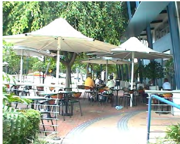
Photograph 6 - Tactile paving free of obstructions
