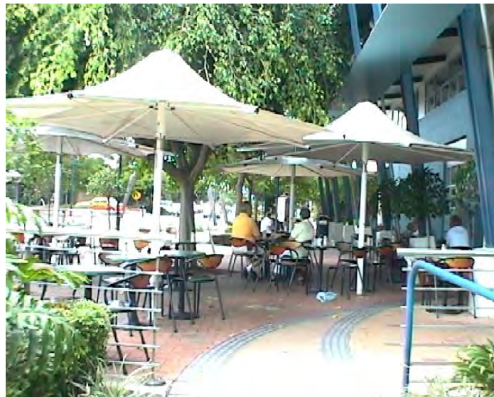
Photograph 6 - Tactile paving free of obstructions
