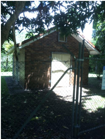
Yerro Creek Water Pump, Dunwich (AHS, 2017).
