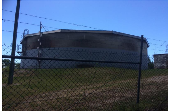
Water Tanks, Dunwich (AHS, 2017).
