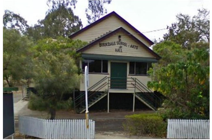
Birkdale School of Arts Hall, Birkdale (RCC, 2013).
