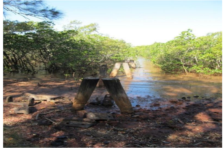
Empire Point Foreshore, Jetty Remnants (RCC, 2013).
