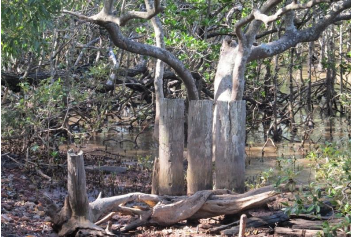
Empire Point Foreshore, Jetty Remnants (RCC, 2013).
