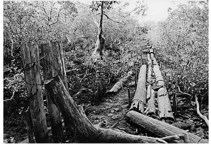
Empire Point Foreshore, Jetty Remnants, c.1995 (RCC, 2013).
