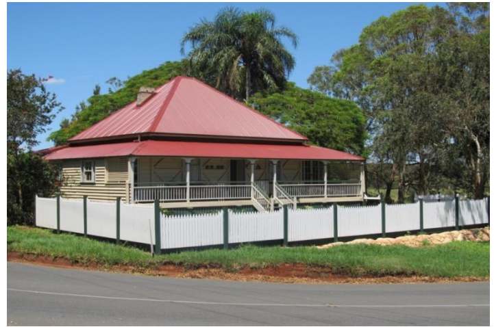
Residential Dwelling, Redland Bay (RCC, 2013).
