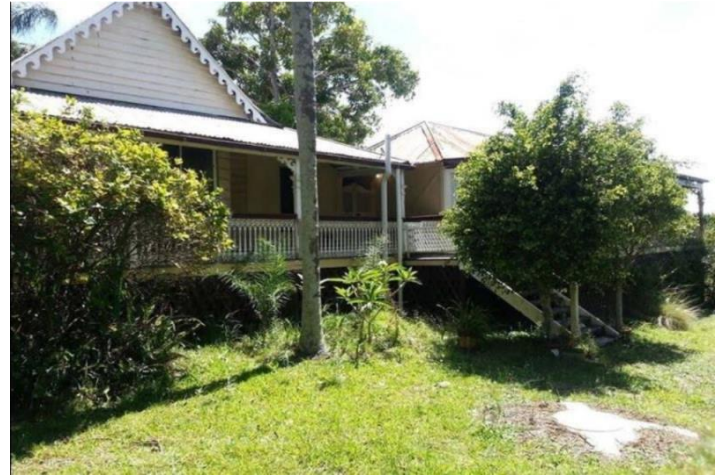
Willard's Farm, Birkdale (RCC, 2016).
