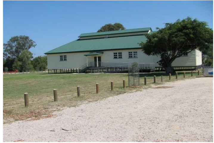
Edgar Harley Pavilion, Cleveland (RCC, 2013).
