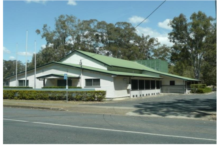
Thorneside Public Hall (RCC, 2013).
