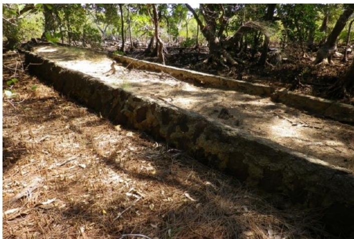
Morton Steps and Jetty, Coochiemudlo Island (RCC, 2013).
