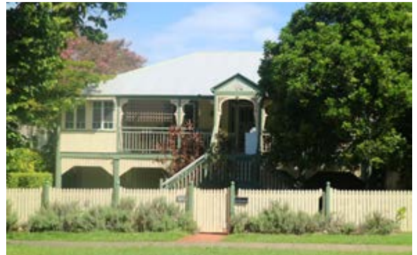
● Direct pedestrian access to the street ● Pitched roof with articulated entrance ● Parking under house or behind building frontage ● House set back from road frontage with landscaping/trees contributing to streetscape
