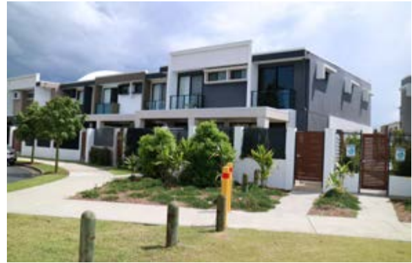
Front doors addressing the street.
