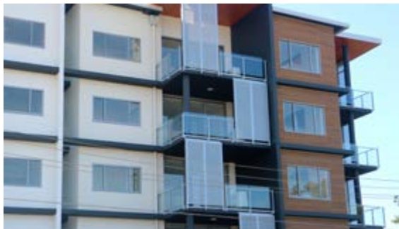
Figure 10 Design includes lattice operable screens, prominent vertical columns, composite timber cladding to the walls and exposed eaves. All units have private open space that achieves natural light. Each unit has dual aspect to promote cross ventilation.
