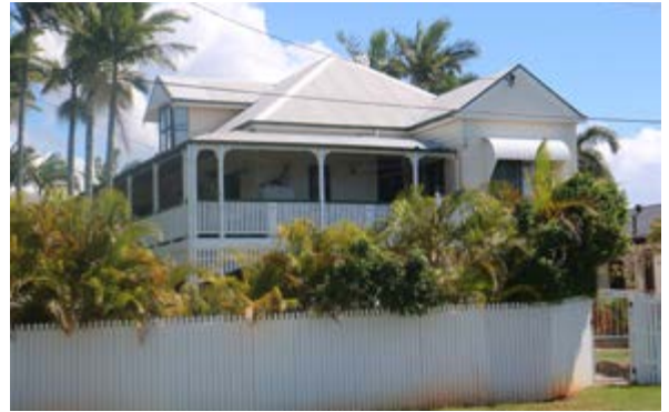
● Addresses both street frontages ● Multiple roof pitches and varying heights ● Projections and recesses in facade ● Outdoor living – wrap around covered balcony
