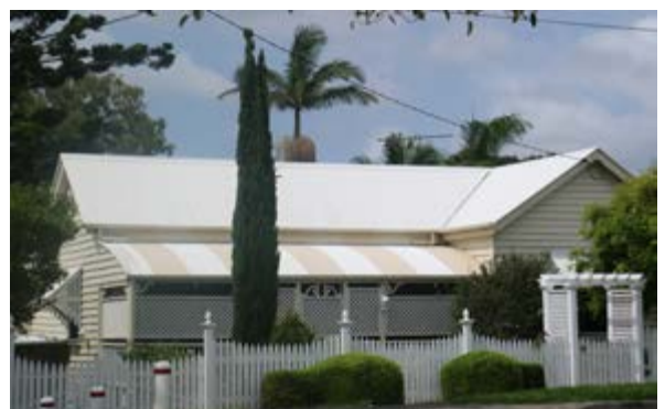
● Bull nose roof on verandah ● Timber picket fence ● Light with materials, timber frame and corrugated iron ● Articulated entrance with Timber arbor ● Landscape strip along frontage
