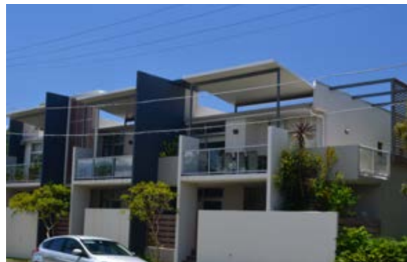
Elevated eaves creates shading and captures cooling breeze plus breeze filtered through screens at entrance and circulation points between the dwelling units.
