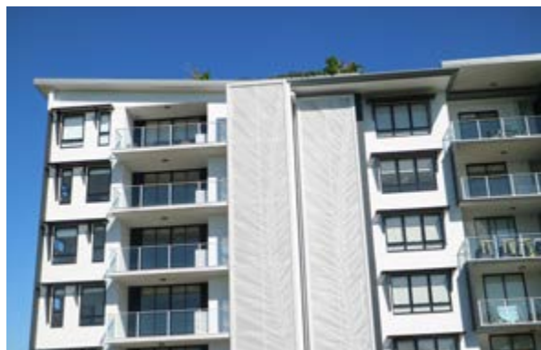
This apartment block has a north eastern aspect. The artistic screening provides a distinct identity and gives vertical emphasis to break up the long facade.
