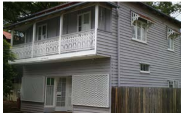
● First floor projection ● Operable windows maximize natural ventilation and prevailing bay breezes ● Chamfer board wall cladding
