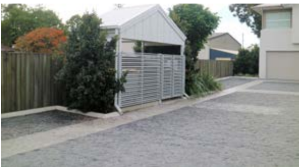
Multiple services screened within the design.
