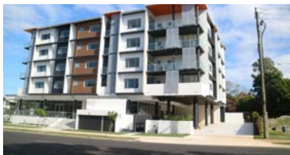
Figure 11 Vehicular access is provided off the secondary road frontage. Car parking is mostly within the basement, with visitor parking in undercroft. Services are screened and incorporated into the overall design.
