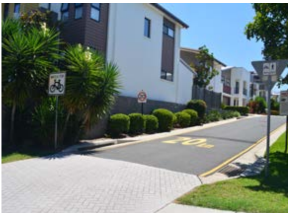
Shared surface clearly delineated by materials and markings
