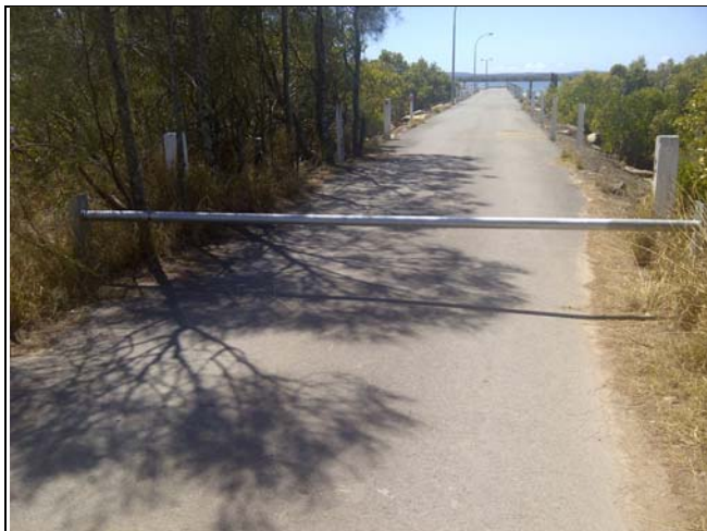
Slip Rail Installed (since replaced by a locked/lay-down bollard)
