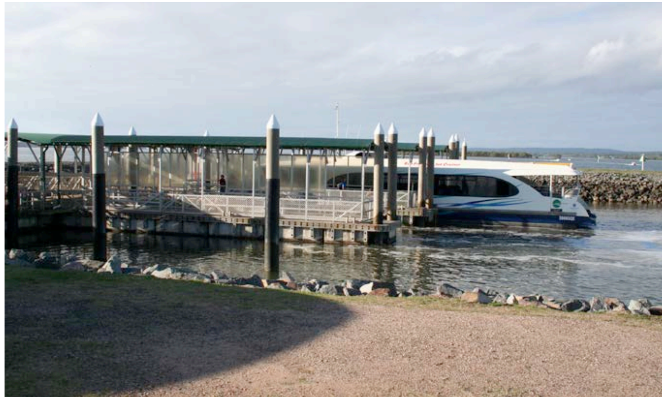
Redland Bay Ferry Terminal
