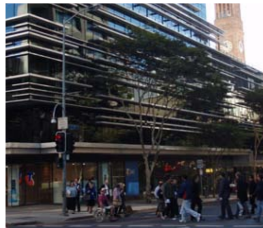
Car park accommodated in podium sleeved with office suites
