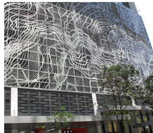
Car park accommodated in podium screened with artwork
