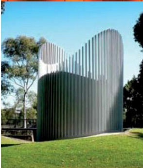
Australian Institute of Architects - Architecture Gallery Transgrid Ventilation Shaft Copyright 2009 http://www.architecture.com.au/awards_search
