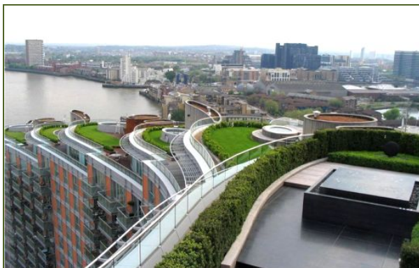
Above: London, New Providence Wharf
