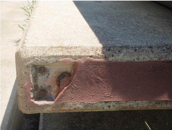
Photo 4 – Top End of Blades Corrosion to Reinforcement
