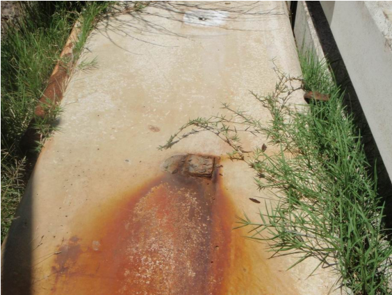
Photo 3 – Corrosion of Fixings
