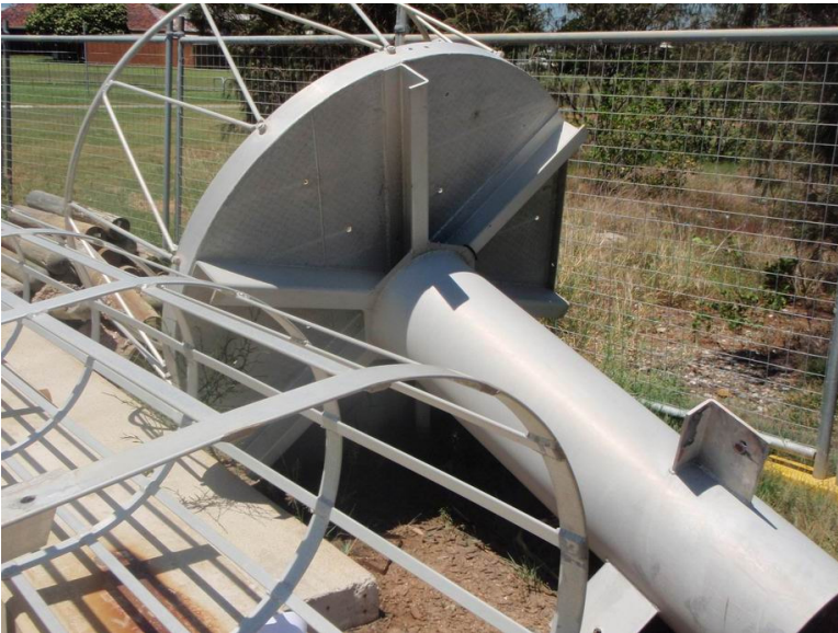
Photo 5 – Structural Steel – Sound Condition
