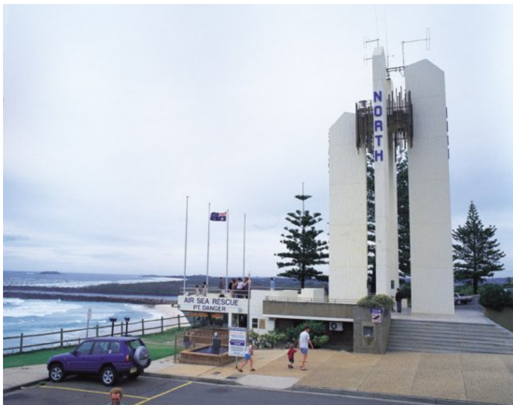
Fig 8: The Point Danger Lighthouse, noting the radial concrete blade structure typology similar to the Cleveland Point lighthouse. Photograph: Annette Flotwell
