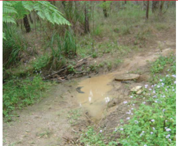
Figure 74: eroded track along watercourse to be closed and rehabilitated
