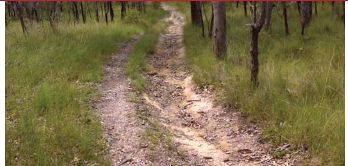
Figure 66: erosion on Magic Track- track can be realigned away from fall line
