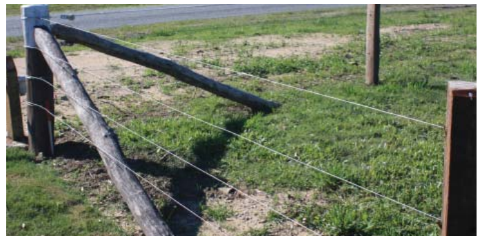
Figure 15: Post and wire 4-strand fence. The picture shows a split post. Corner tensioning can be achieved by use of simple logs
