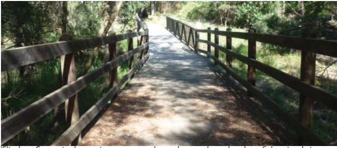
Flinders Street is the main access track on the northern border of the site. It is primarily a concrete pathway, and forms a part of the Cleveland-Capalaba major cycle and pedestrian trunk connection
