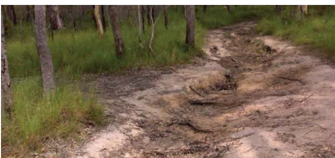
Fire Control Trails within the site are eroded in places
