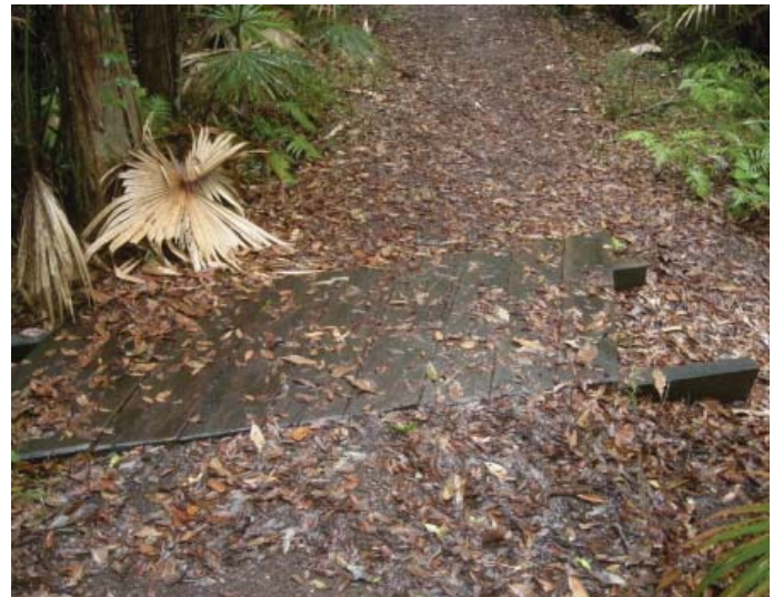
Figure 47: A covered cross drain
