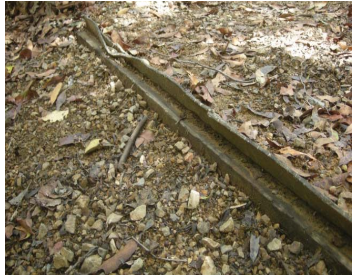
Figure 46: Timber with rubber water bars. Regular maintenance is required to ensure the soil under which the timber is buried does not become exposed (as has occurred in the above photo) as such exposure creates a hazard or cyclists
