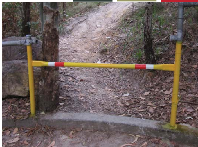
Figure 72: Existing entry has severe erosion above gate. Close entry and path and rehabilitate. Realign path away from Creek corridor to join Sewer/ Bondi Tracks entrance
