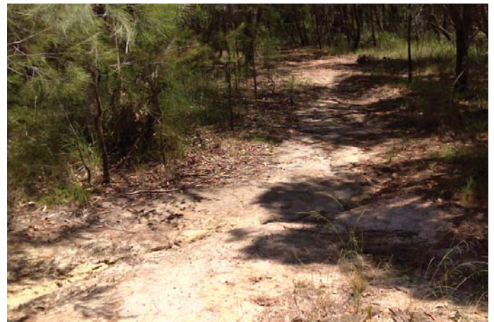
Figure 63: Water Track has good tree coverage, however is poorly designed. The cleared width allows for vehicles however the track width appears narrower due to leaf litter
