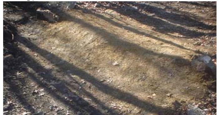
Figure 55: rolling grade dips are low maintenance, attractive erosion control measures
