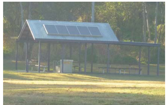
Figure 32: Picnic shelter with solar panels for lighting is a sustainable solution to energy use (Colmslie Park Brisbane)
