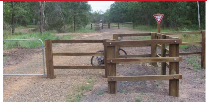
Figure 13: Brisbane Valley Rail Trail at Coominya. Pedestrian/Bicycle gate where cyclists can negotiate without having to dismount (though they still need to slow down). Access for trail bikes is prevented due to narrowness of openings
