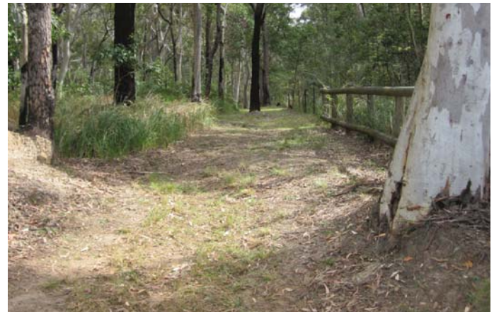
Figure 60: existing firetrail from Clarke Street to become Clarke Reserve Entry Track, with smooth graded compressed earth surface.
