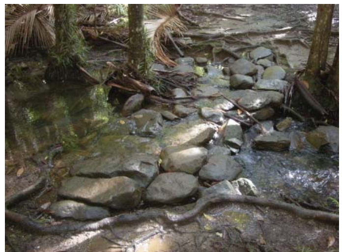
Figure 48: Stepping stones. The stepping stones are strategically placed along the stream to form the trail
