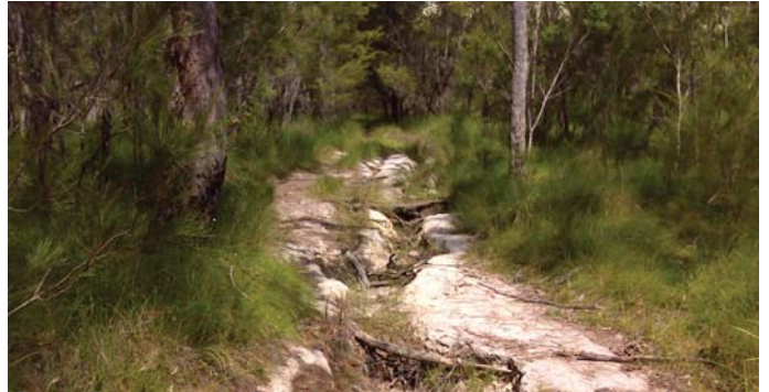
Figure 67: eroded existing firetrack to become Lower Magic. It can be redesigned with tree roots, water erosion control measures as riding obstacles
