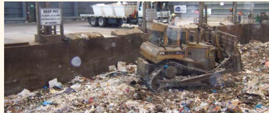
Examples of transfer station push pits
