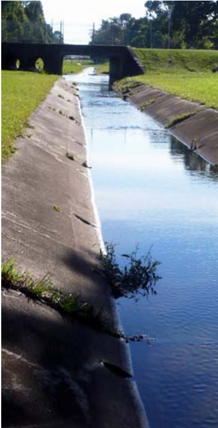
Existing culvert section
