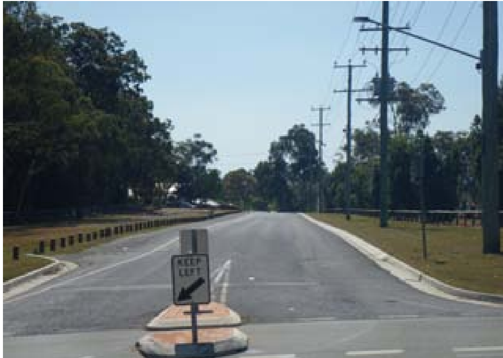
Clarke Street Existing Streetscape
