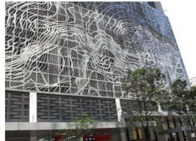
Car park accommodated in podium screened with artwork
