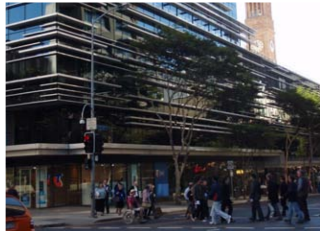
Car park accommodated in podium sleeved with office suites
