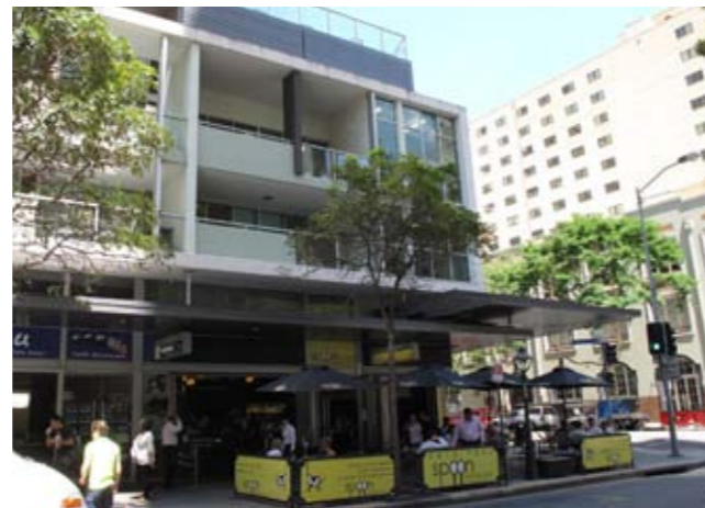
Residential studios sleeving podium car park provide natural surveillance of the adjacent street
